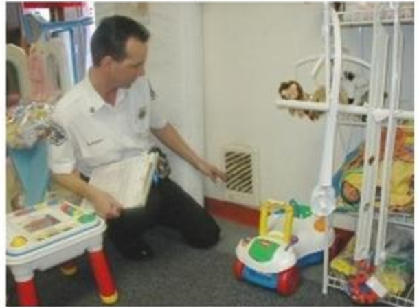
Deputy Fire Marshal Chad Lawry assisted a Vancouver business with the identification and replacement of a recalled Cadet in-wall heater.
